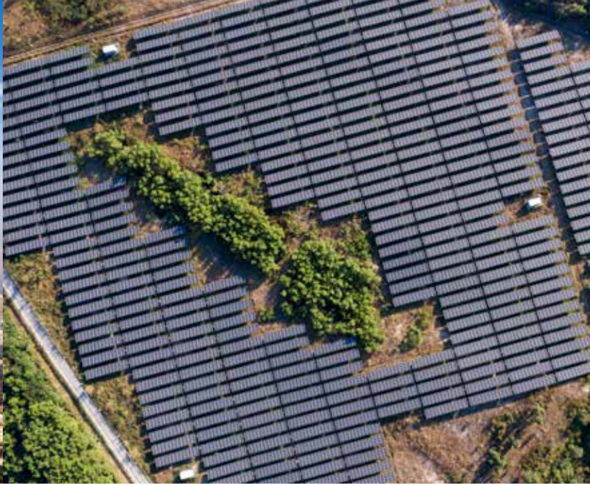
Aerial Inspections of Solar Installation near Pushkar, Rajasthan
