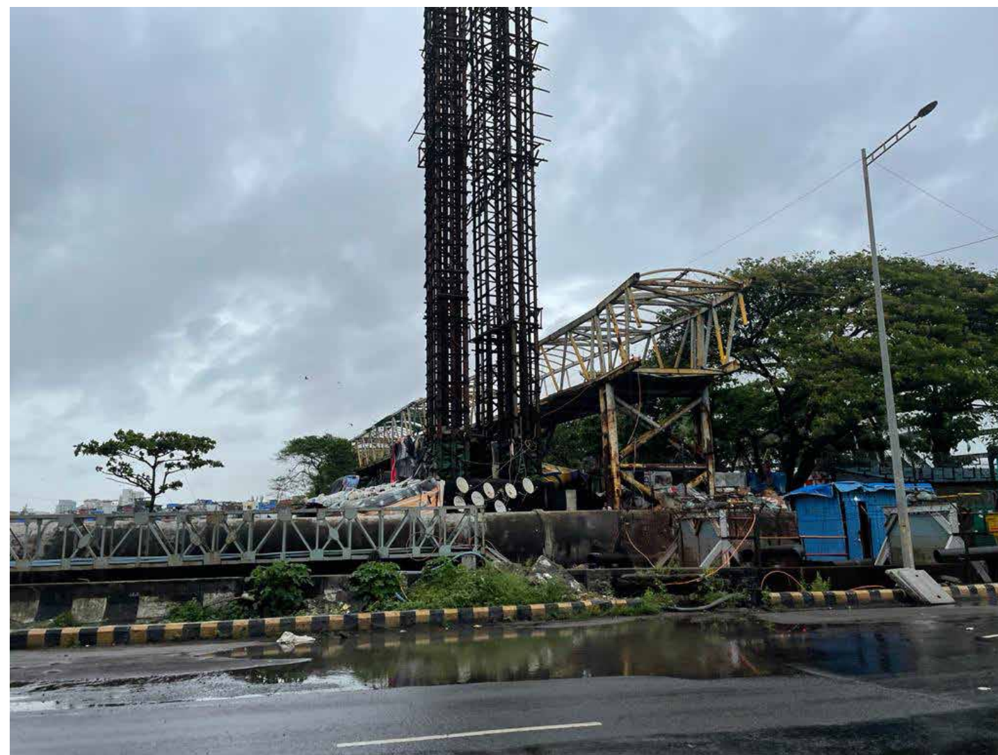
1 Opposite Hotel Radisson at Egmore, Chennai, India
